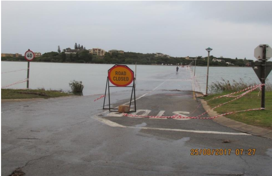
Plate 10 Berm overwash shown in Plate 8 resulted in the causeway overtopping with seawater. Zero freshwater inflow to the estuary occurred around this time, so that salinity levels in the estuary would remain at 35 or higher. High rates of evaporation would rapidly result in hypersaline conditions developing in the estuary as the estuary closed again within 48 hrs. Photograph from Hennie Swanevelder – Department of Economic Development and Environmental Affairs.
