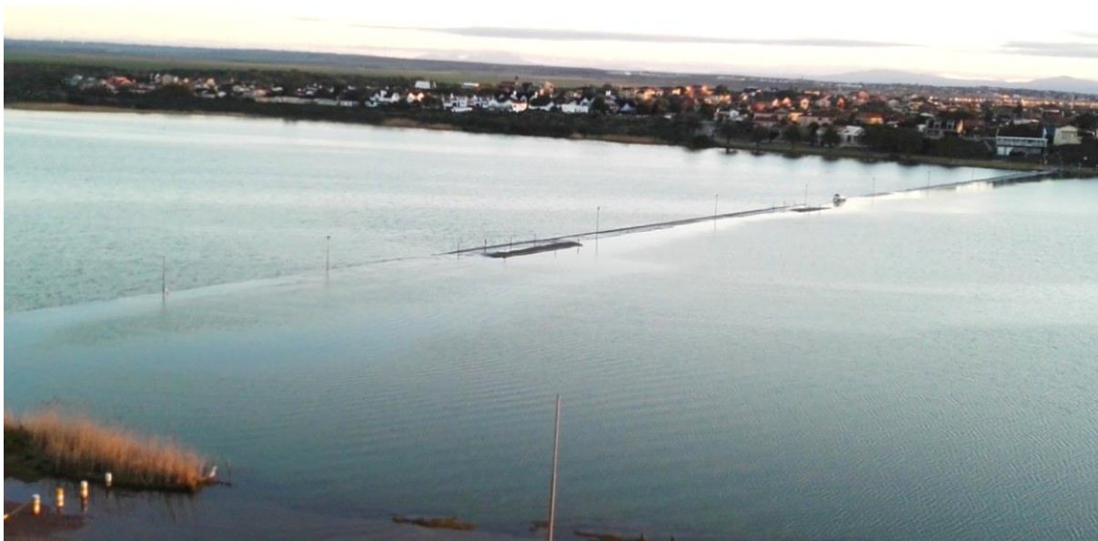
Plate 11 Overtopping of the berm causes significant damage to vehicles (electrical issues included) and puts life at risk (vehicles sliding off the causeway, pedestrians crossing on foot), particularly under windy conditions. Both photos demonstrate the undulatory nature of the roadway.
