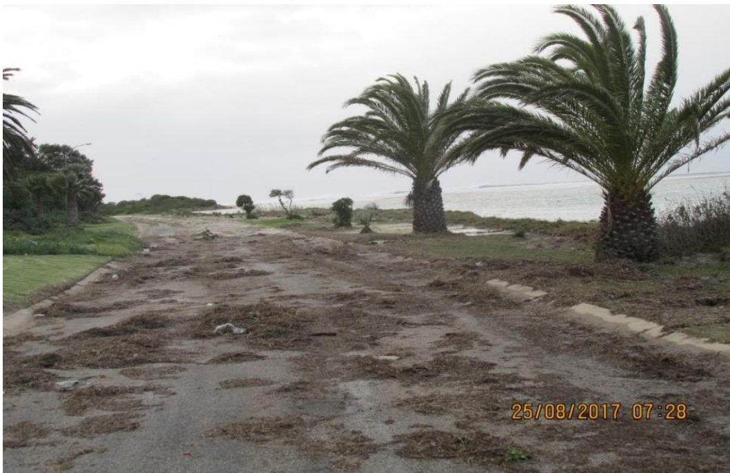
Plate 9 Berm overwash shown in Plate 8 deposited large quantities of flotsam on the Aston Bay road running parallel to the estuary. Photograph from Hennie Swanevelder – Department of Economic Development and Environmental Affairs.
