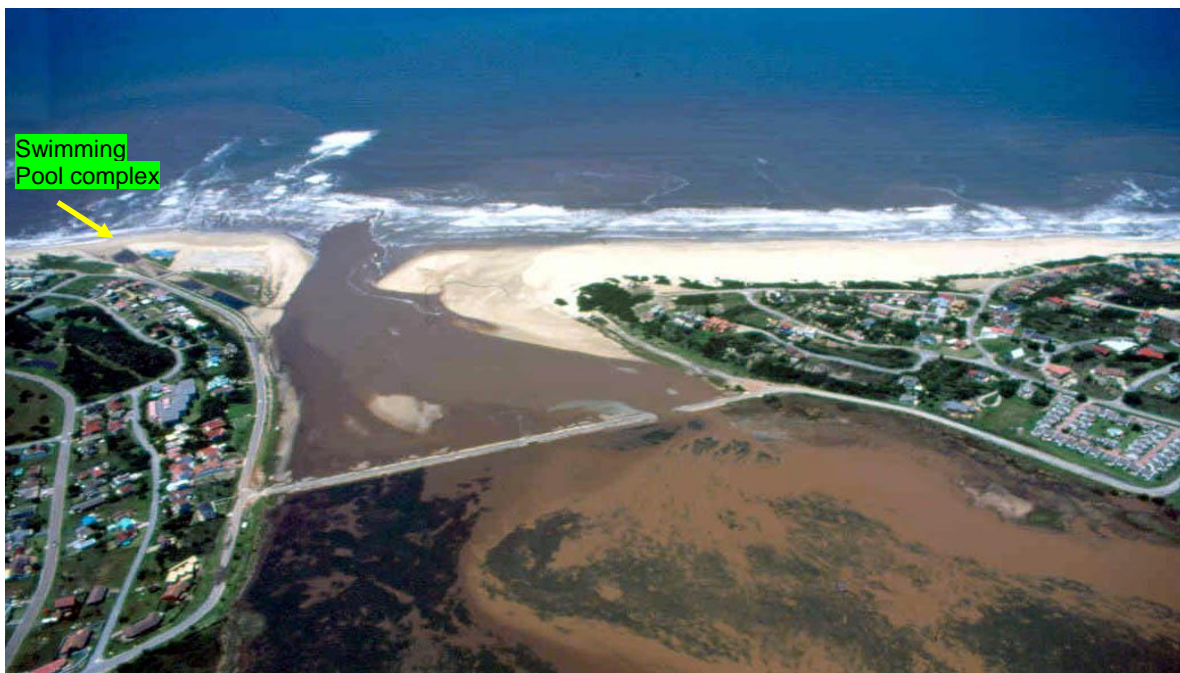
Plate 4 At the time of this photograph (mid 1980's), the original rubble causeway had been breached and floodwaters eroded a relatively deep and wide channel. The photograph also shows a plume of discoloured estuarine water radiating from the mouth – refer to Figure 7 (Photograph from T Wooldridge).
